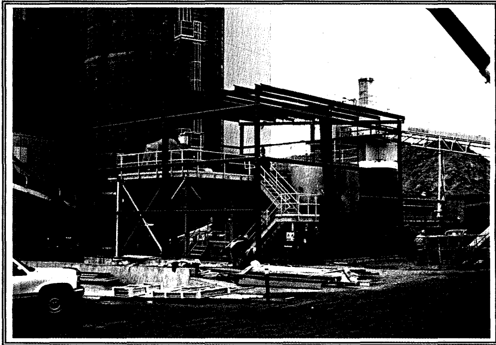
Figure 6: Process water fines handling building under construction.
