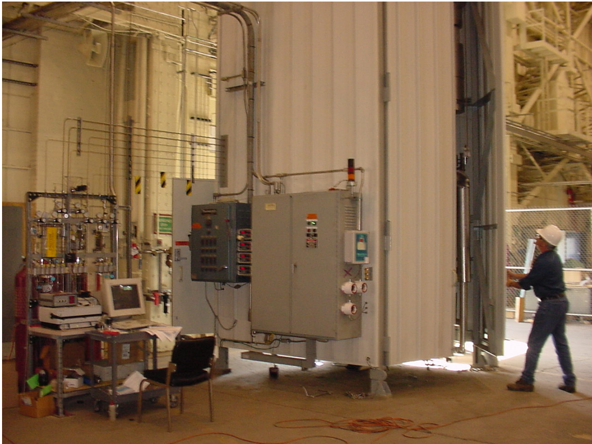
Long Tube Tester Pilot Plant Facility
