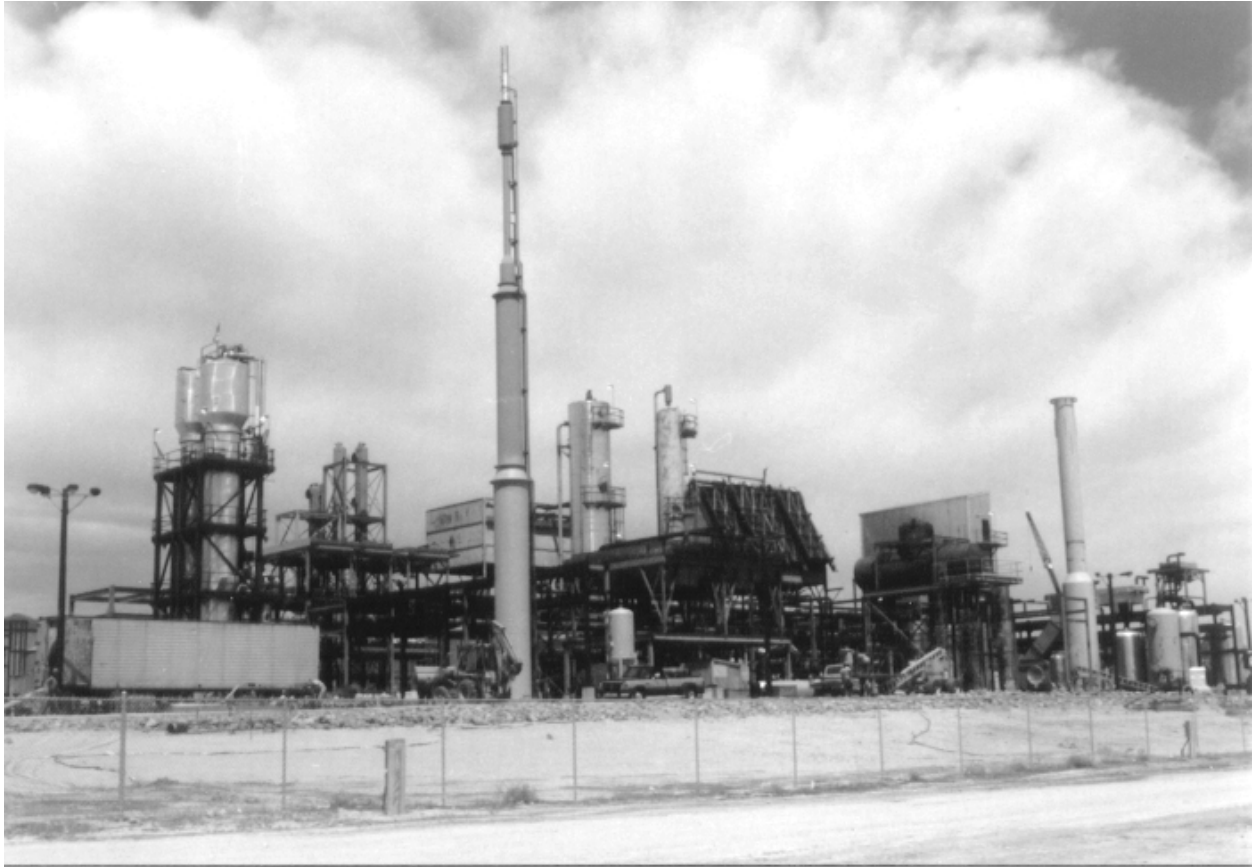
Commercial scale gas-to-liquids plant in Pueblo, Colorado fueled by landfill methane gas (1992) (Photo courtesy of Rentech, Inc.)
