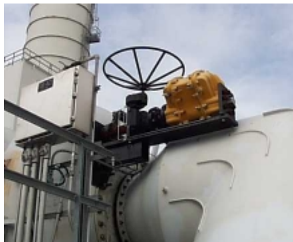
Figure 5.1.1B: Close-up of a Newly Installed Guide Vane Actuator
