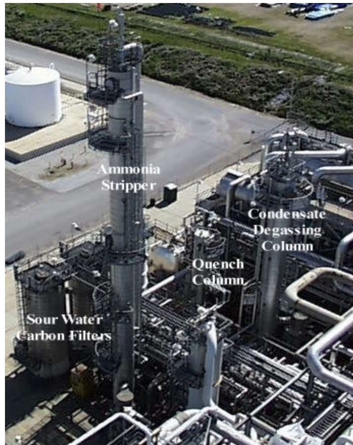
Figure 5.3.13A: Sour Water Treatment System Major Equipment
