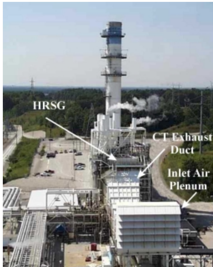
Figure 5.4.1A: Combustion Turbine
