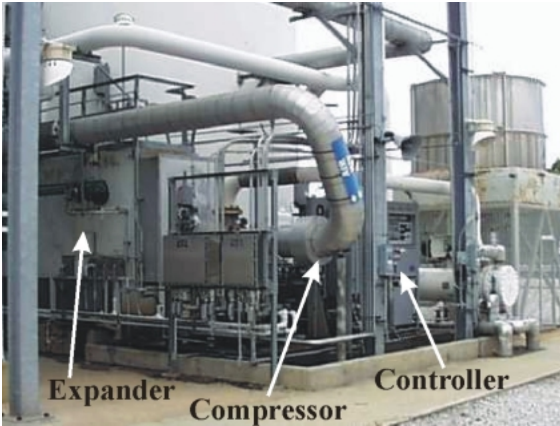
Figure 5.1.4B: Compressor/Expander Skid
