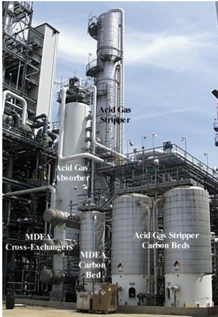
Figure 5.3.11A: Acid Gas Removal System Major Equipment
