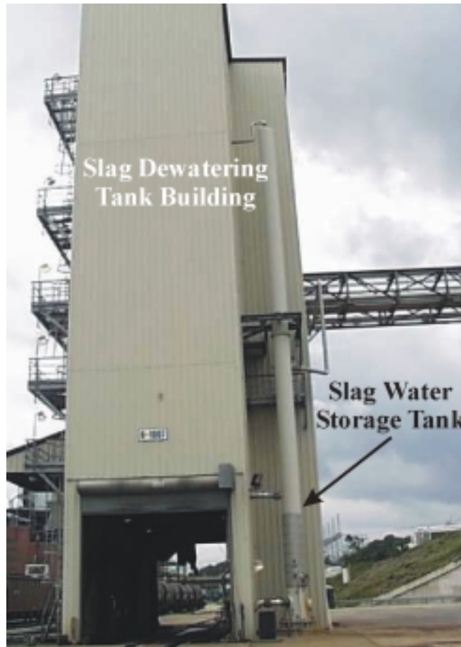
Figure 5.3.4A: Slag Dewatering Tank Building and Slag Water Storage Tank
