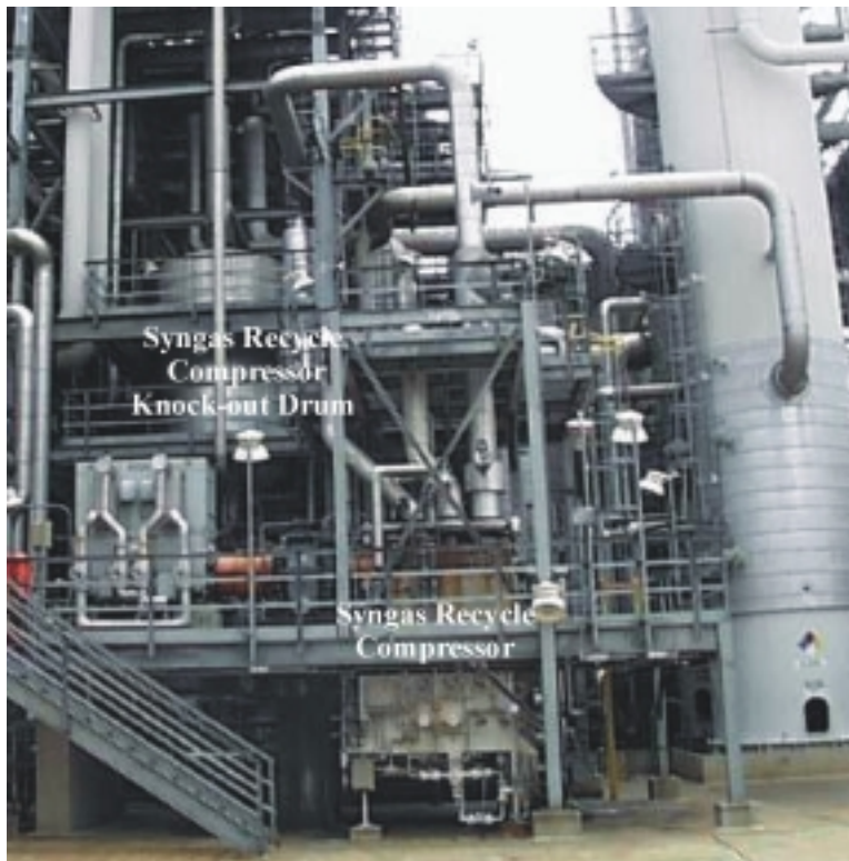
Figure 5.3.9B: Syngas Recycle Compressor and Knockout Drum
