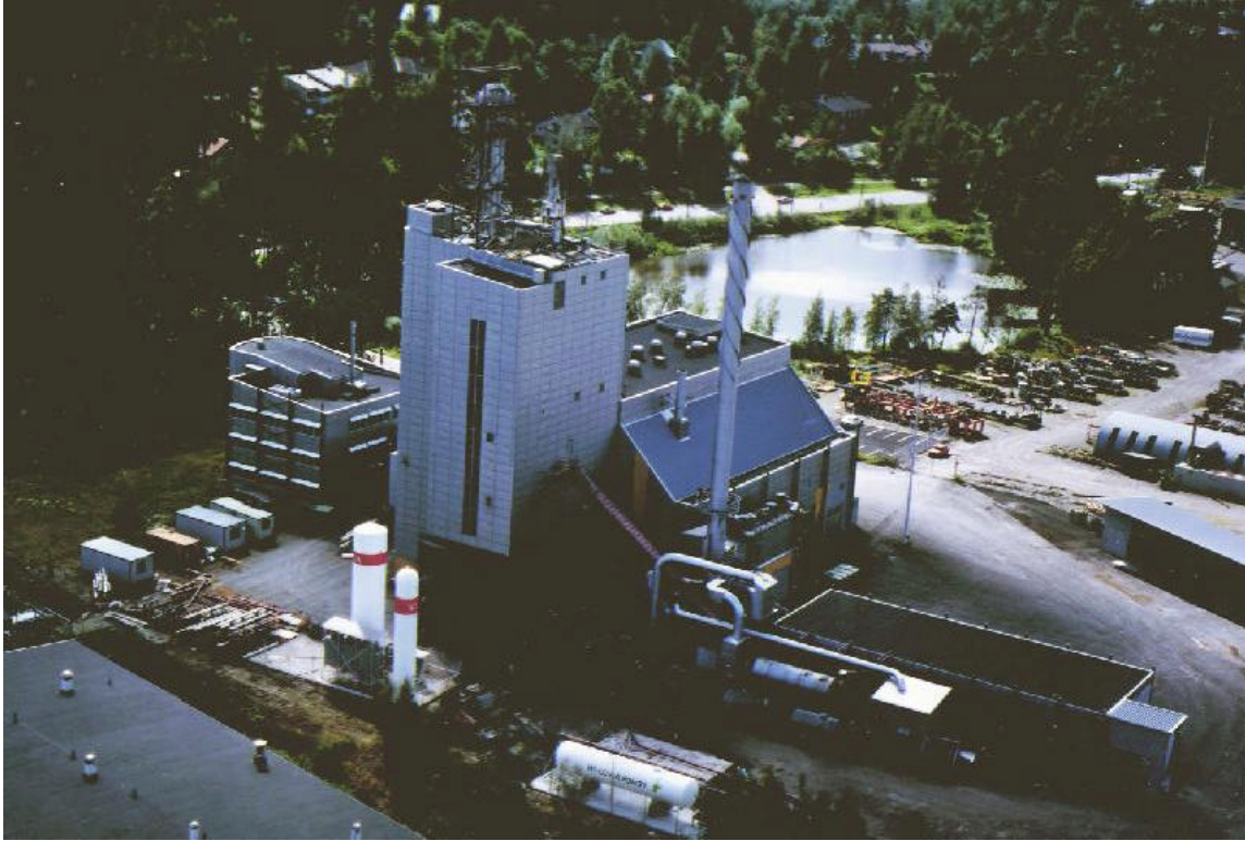
Figure 29. Picture of the Gasification Demonstration Plant in Tampere, Finland (Courtesy of Carbona)
