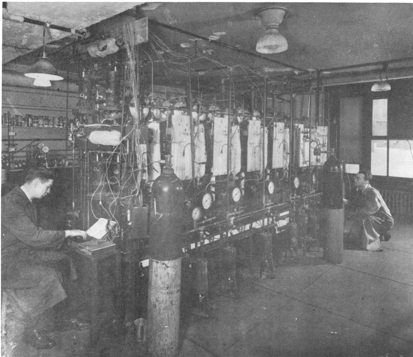
Figure 34.- Catalyst testing units. Front view.
