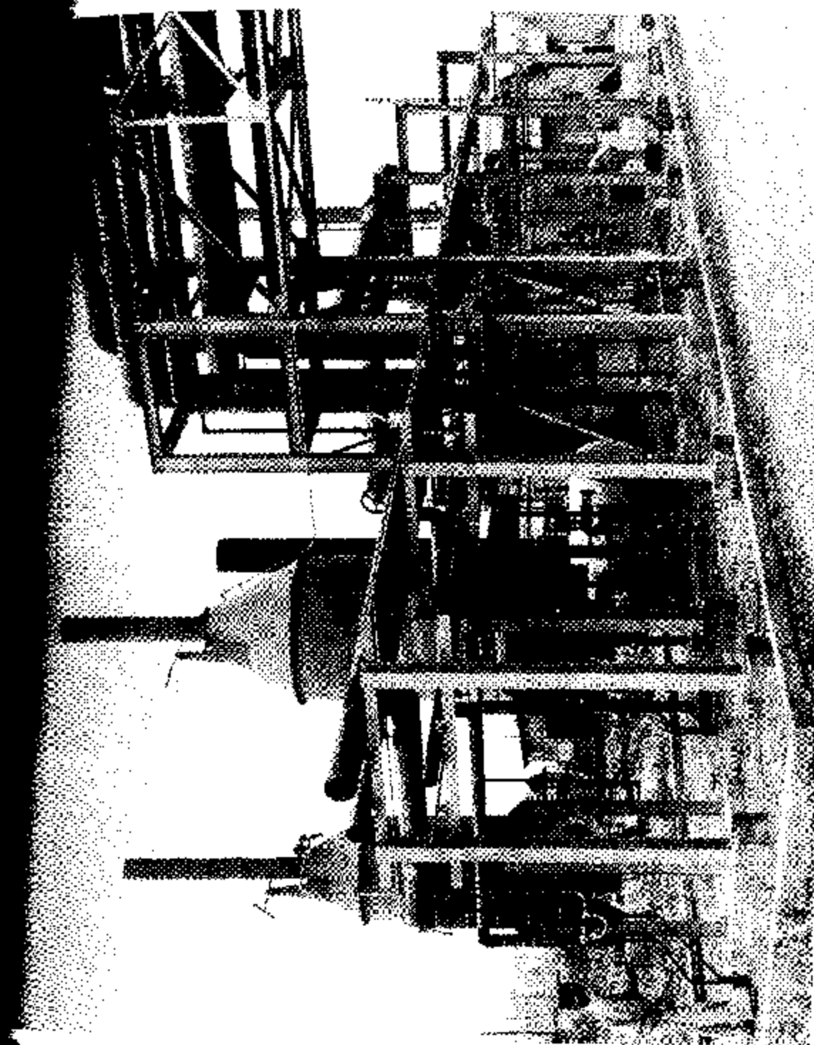
Figure 19. - Gas-fired heaters for preheating feed streams to synthesis and distillation units, Gas-Synthesis Demonstration Plant.
