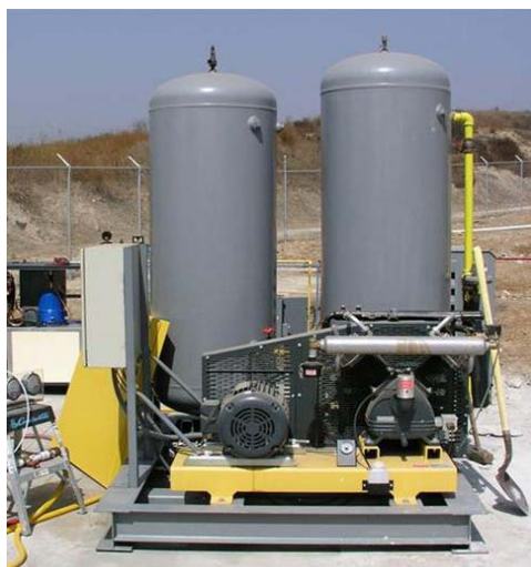
Figure 19. High-pressure air feeding system: high pressure and low-pressure receiver tanks.
