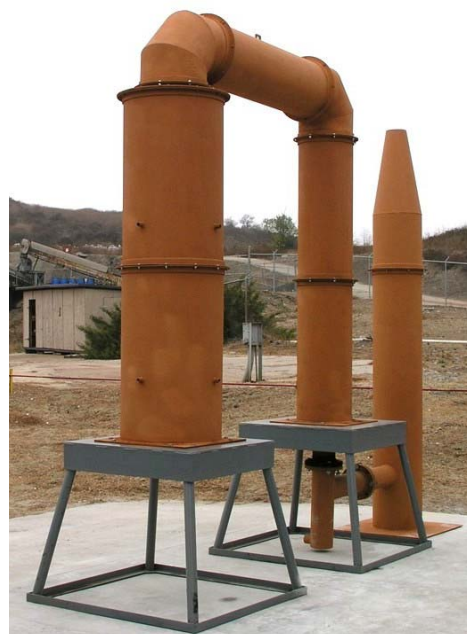
Figure 22. Emissions control system: afterburner, quench, and scrubber in series.
