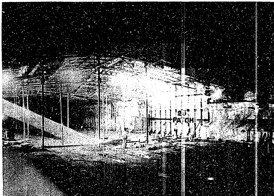
Figure 12 Damage from Bomb No. 2. Temporary repairs in progress to make flight deck watertight.
