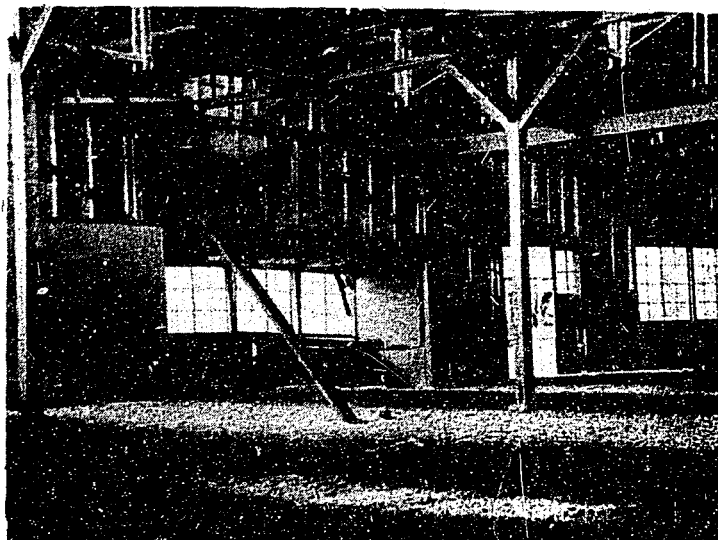
Figure 7 INTERIOR OF TIMBER STRUCTURE SHOWING UNEQUAL SETTLEMENT OF FOUNDATION UNDER END WALL OF BUILDING Note detail of brackets at column head. See next photo for closeup of damage to concrete slabs in center background.
