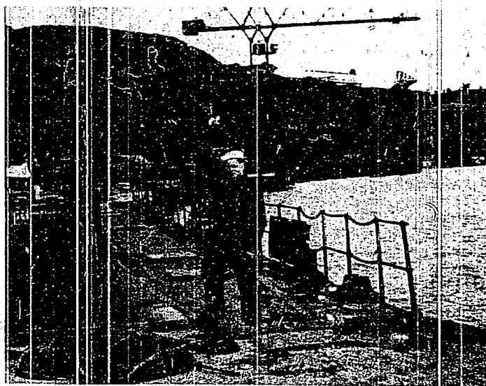
Figure 10 CAISSON, NO. 4 DRY DOCK (Framework of gantry crane supports at No. 2 building slip, visible in background.)
